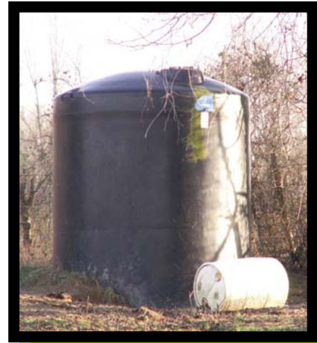
Water Tank Supplied by Solar Powered Pump
