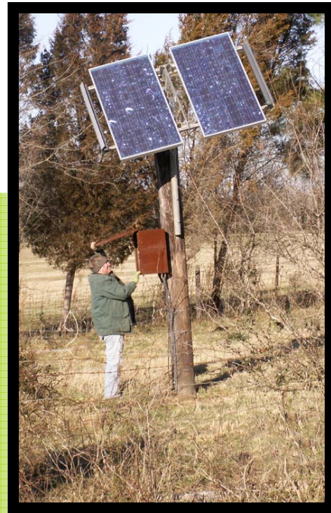
Solar Powered Panels for Water Pump
